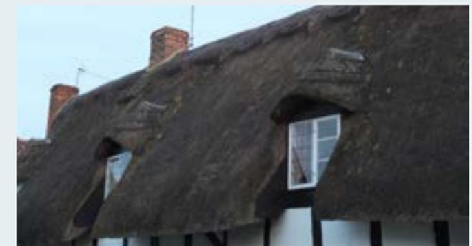
The pitch of the roof is usually at 45 degrees or more to allow water to run off easily. The wire netting used is not to hold the thatch in place but to stop birds (and other creatures) from making nests.
